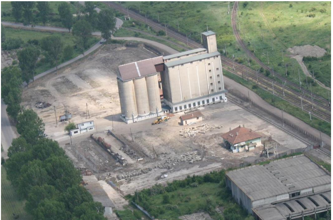
Silo FirstFarms East Romania
